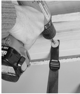
figure 6.1 Attach your four straps to the floor joist making sure that you attach thru the washers and the grommets.
