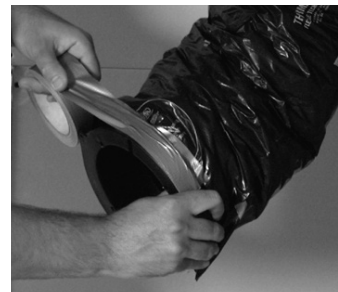
figure 7.3 Finish by taping the vapor barrier to the collar to insure proper seal.
