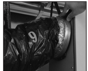
figure 7.4 Slide collar on the unit.
