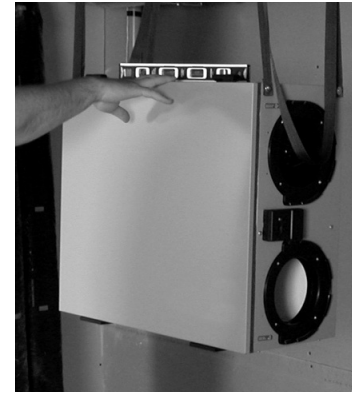
figure 6.3 When completing the procedure make sure that the HRV or ERV is leveled.
