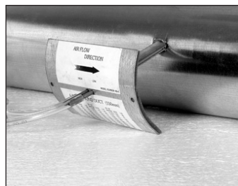
Inserting Air flow grid in duct
