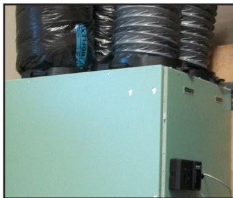
figure 7.4 Slide collar on the unit.
