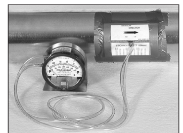
Seal Air flow grid in duct with duct tape.
