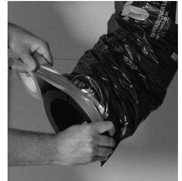
figure 7.3 Finish by taping the duct on the collar.
