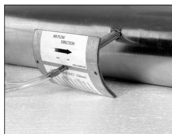
Inserting Air flow grid in duct
