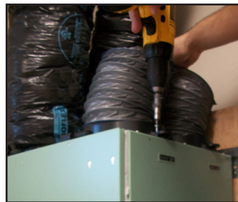
Figure 7.5 Fix and secure the collars to the HRV/ERV with the #10 x 1/4" screws, supplied in kit.
