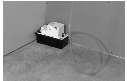
figure 8.2 Use a condensate pump if you don't have access to a drain.
