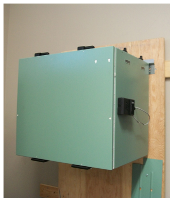
figure 6.2 Hang HRV/ERV to wall mounting bracket.
