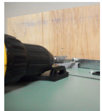
figure 6.4 Proceed to secure HRV/ERV to bracket with the two #8 x 3/8" screws.
