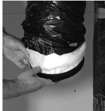
figure 7.2 Insert insulation inside the collar.
