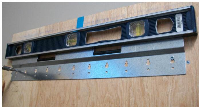
figure 6.1 Installation of the wall bracket. Secure with two #10 x 1 1/4" screws.
